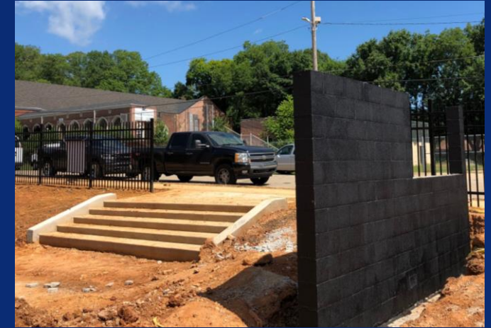
North Steps and Monument Sign Install (in progress)
