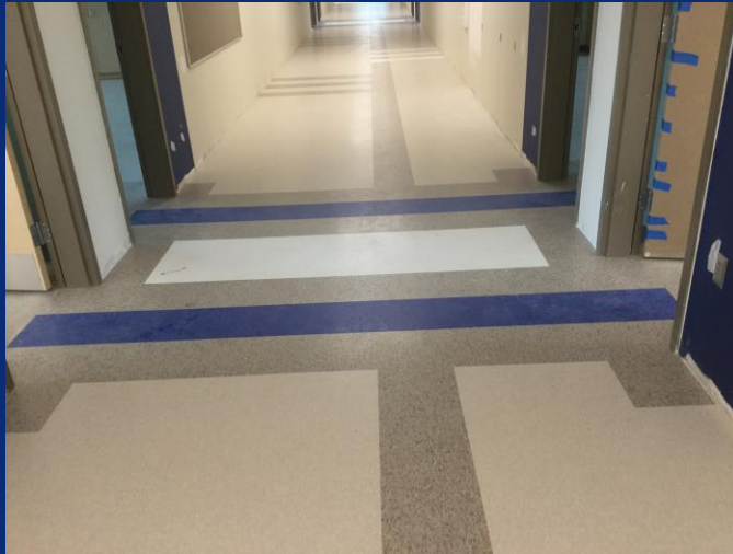
Third Floor Corridor VCT Install
