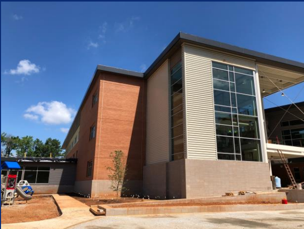
South Stair Tower Metal Panel and Curtainwall Install
