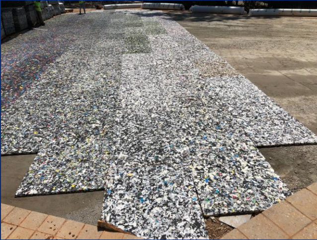
Turf Playfield Foam Install
