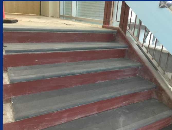
South Stair Precast Tread Install
