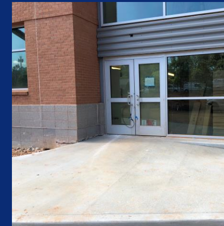
West Stair Concrete Sidewalk Poured
