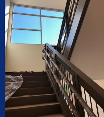
West Stair Paint
