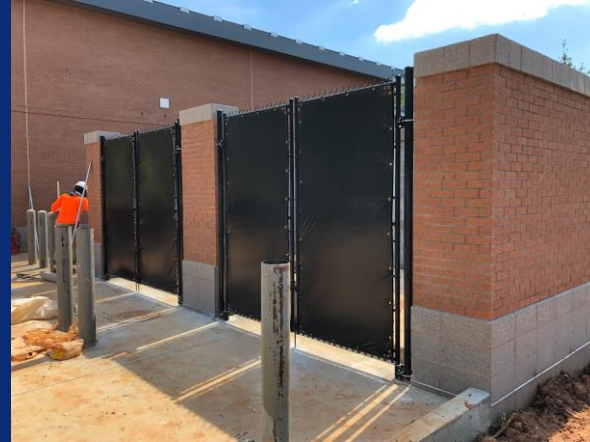
Dumpster Pad Gates Install
